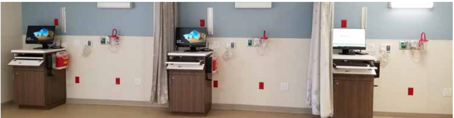
Surgical Center Equipment Procurement and Set-up
